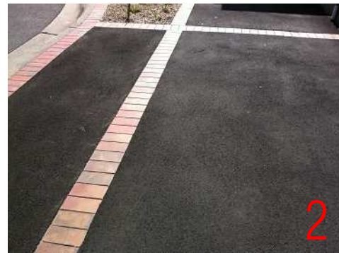
Asphalt paving with brick banding
